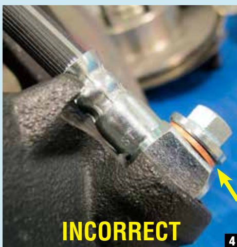
4. Installed backwards, as shown, the shoulder of the hose fitting will come in contact with the caliper, causing the banjo to crush the compression washer at an angle, ultimately leading to fluid leaks. (photo 4)
